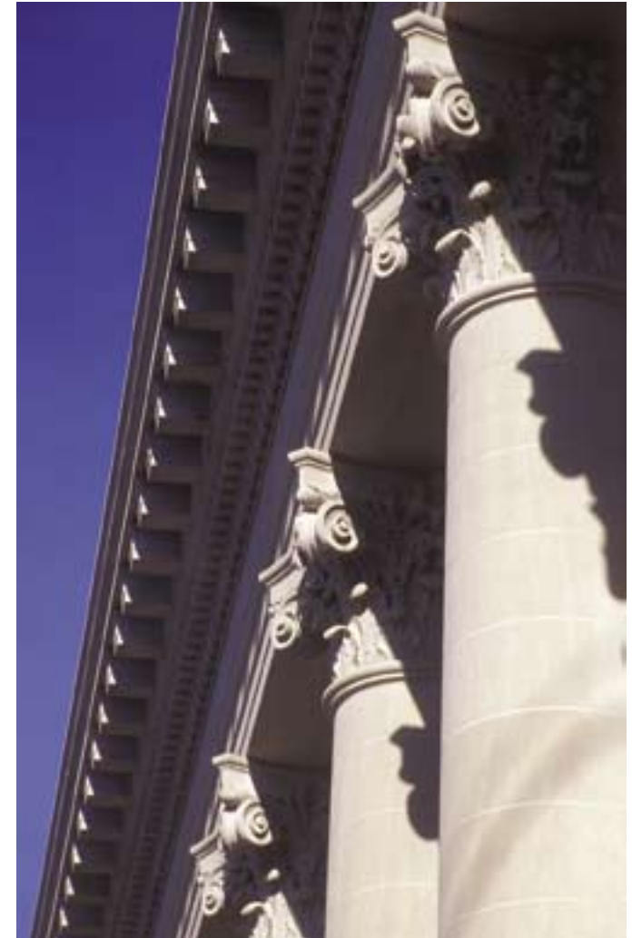
Pillar detail of the Banner Bank Building. Downtown Walla Walla.
